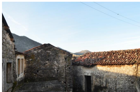
Figure 6. Roofs in village Godinje
